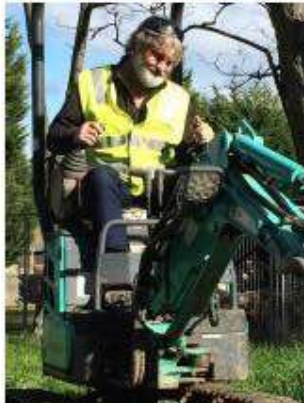
Dave digging the electrical trench at the Men's Shed.
